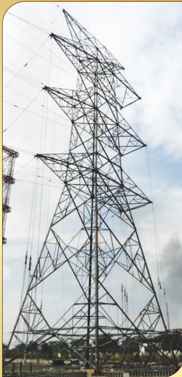
400 kV D/C TOWER FOR KENYA ELECTRICITY TRANSMISSION CO. LTD.
