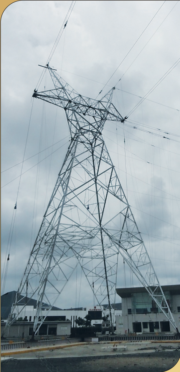
500 kV HVDC BI-POLAR TOWER FOR AECOM CO. CANADA
