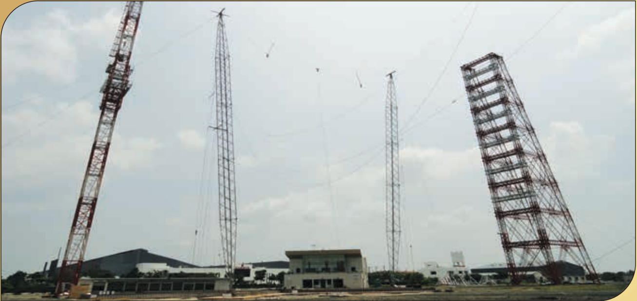
735 KV S/C CROSS-ROPE CHAINNETTE TYPE GUYED TOWER FOR HYDRO QUEBEC, CANADA
